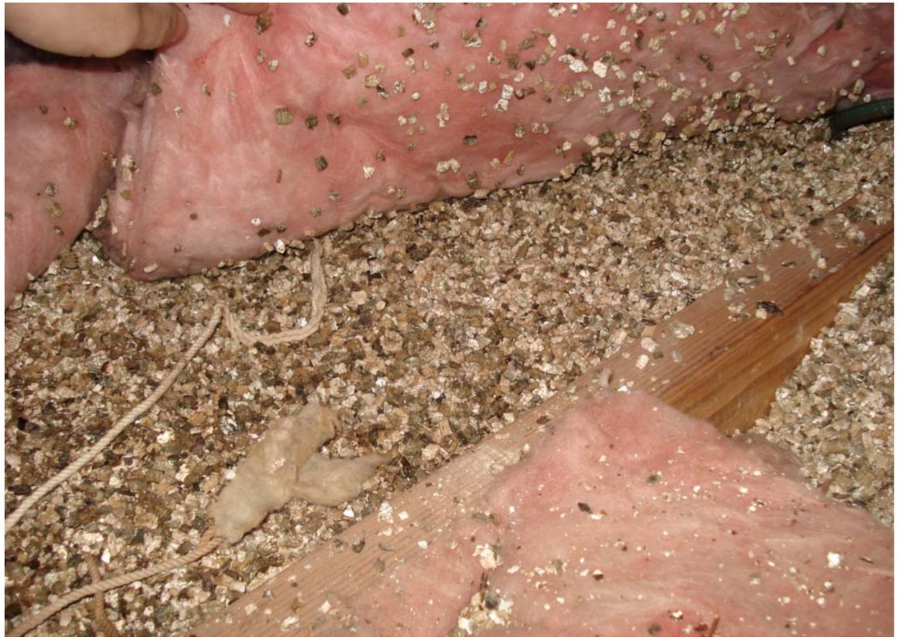
*Vermiculite insulation in an attic, hidden under fiberglass batt insulation, a common application.*
